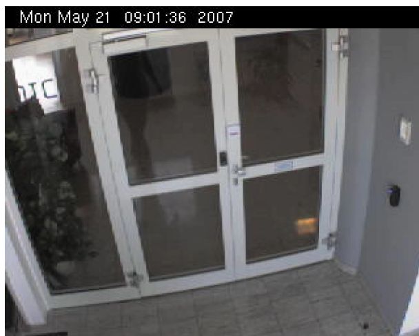
Figure 1. A case access point: the door opens when two sensors on the right side confirm the identity of the acceding person. The upper sensor is an identity card reader and the lower a fingerprint reader.
