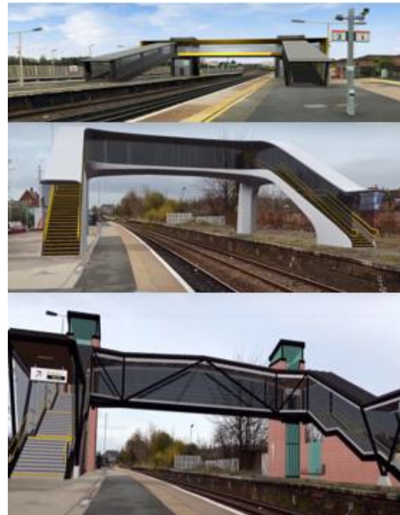
Figure 8: Railway footbridge alternatives designed by AR_BIM.
