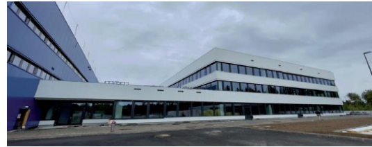
Figure 16: Industrial Building using AR.
