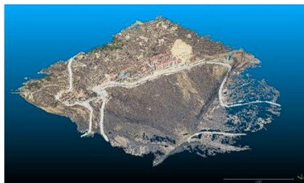
Figure 10: Matching point cloud data for construction site of a certain intelligent building project
