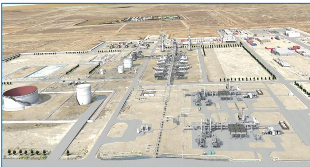
Figure 20: Oilfield pipeline and facilities overview.
